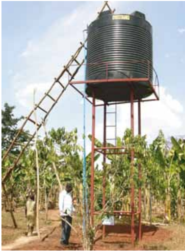
Wassertank 10'000 Liter, Grundwasserpumpe 55 Liter/min
